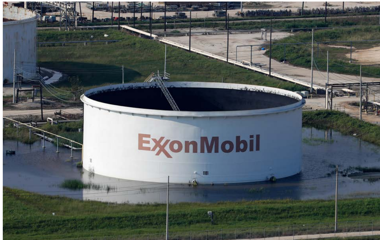
A FLOODED EXXON MOBIL HOLDING TANK IN HOUSTON FOLLOWING THE RECORD FLOODING FROM HURRICANE HARVEY
